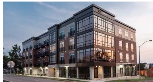
318 E 3rd St: 35-unit multifamily development opened in 2021
